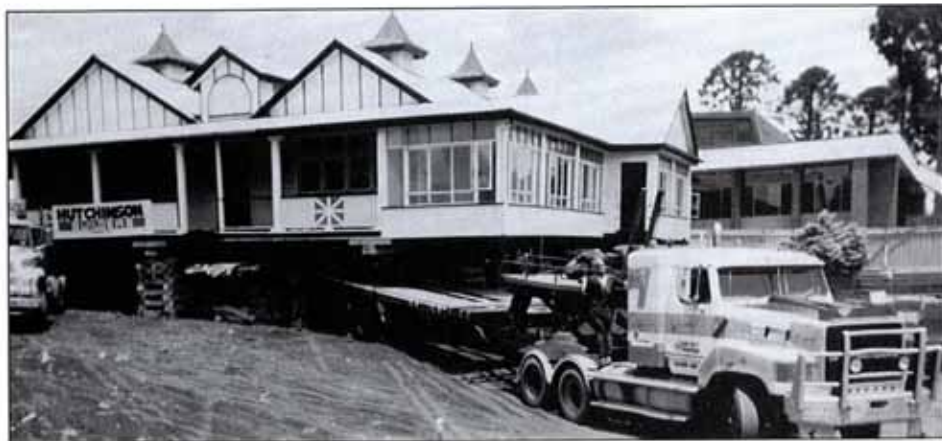
One of Fairholme College's original classrooms gets a helping hand from Hutchies and Transtate House Removals for a whole new lease on life as the top storey of the College's new Performing Arts complex.
